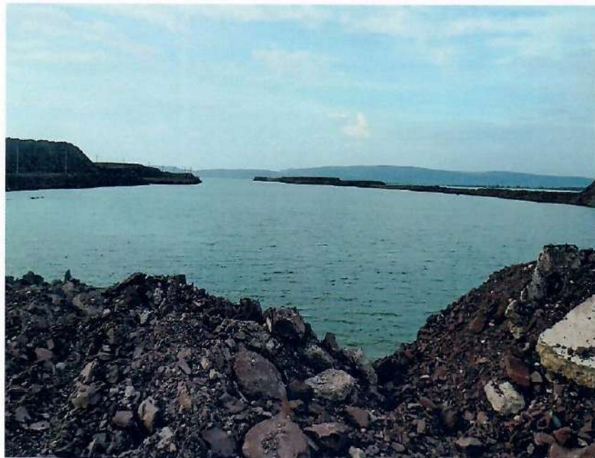
P1: View of Upstream View of the Approach Channel
